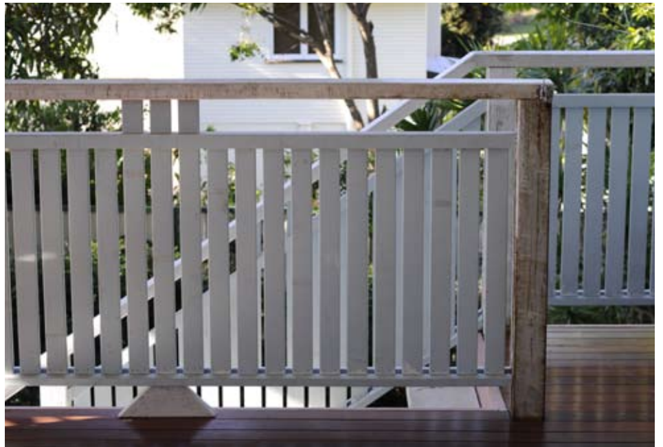
Weakened anchors for balustrades could cause them to fail if people lean against them
